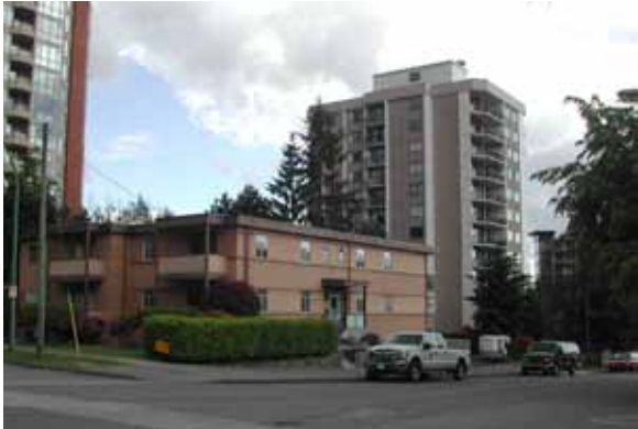
A small apartment building (748 Chesterfield) and the high-rise on the right (701 West Victoria Park), sit on the former Garden Court site. Sharon Proctor photo.
