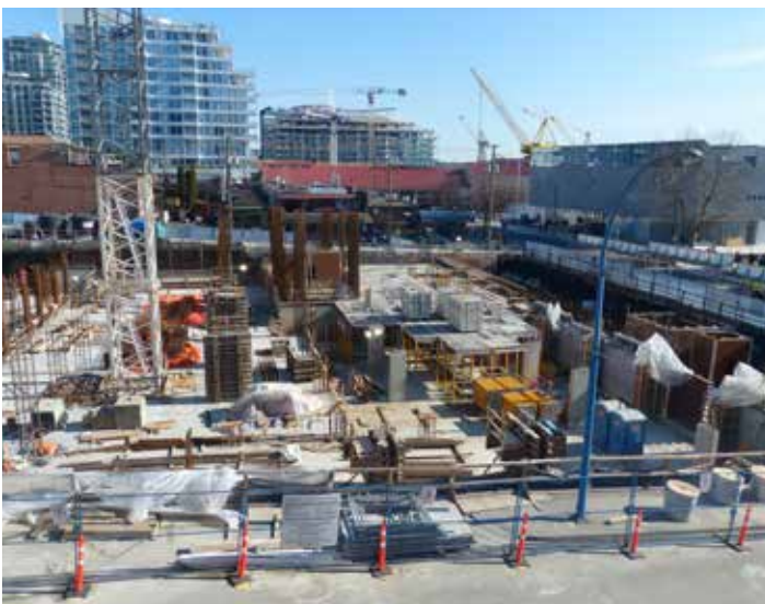
Construction progress, March 2018
